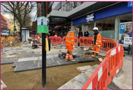
Old Marylebone Road repaved and resurfaced by TfL following lobbying by the BID.
