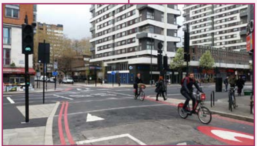
C27 Burwood/Harrowby junction improvements completed.
