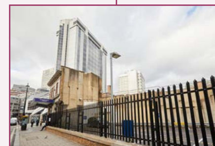
Chapel Street lighting and safety improvements completed.
