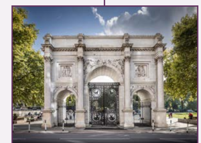
Marble Arch restoration is completed.
