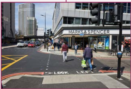
Side road crossings completed.
