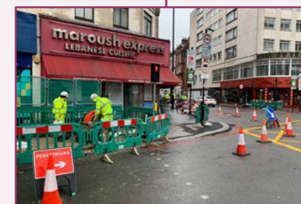
Work starts on site to create side road crossings.
