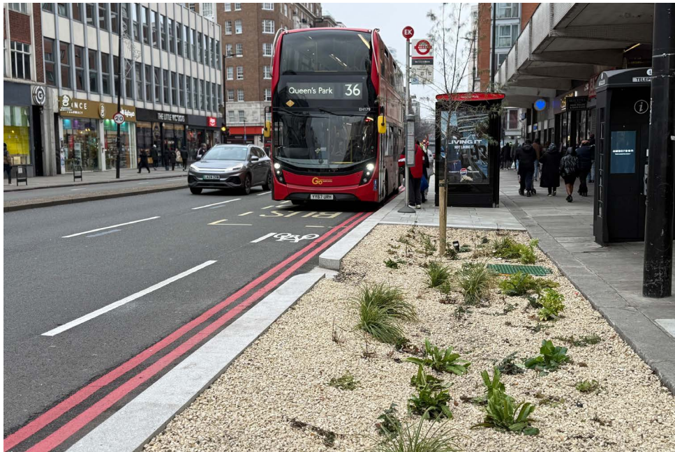
One of the new rain gardens on Edgware Road, helping to prevent surface water flooding.
